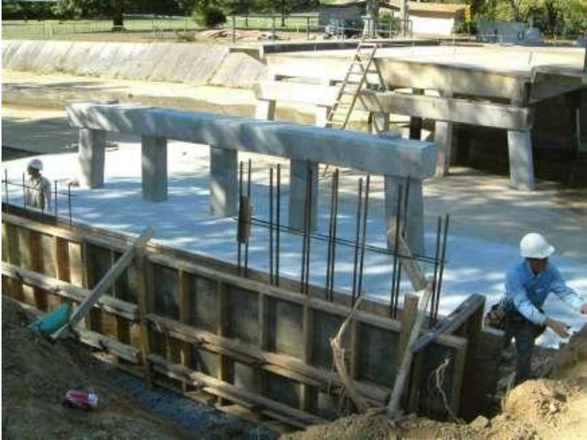
Figure 2-3: Widening of the Lily Flagg Bridge, October 16, 2003.
