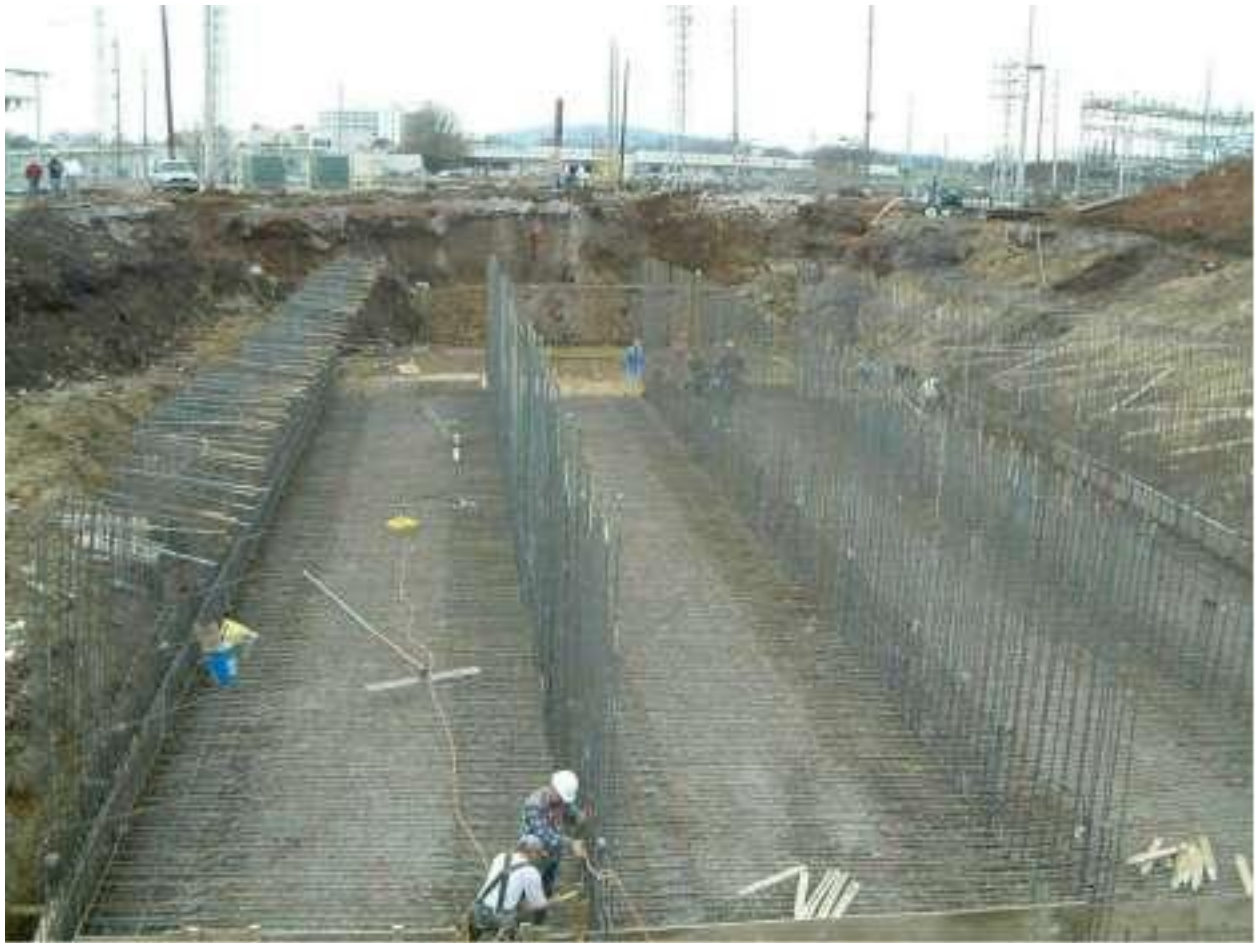
Figure 2-4: New Fagan Creek culvert under construction, December 12, 2003
